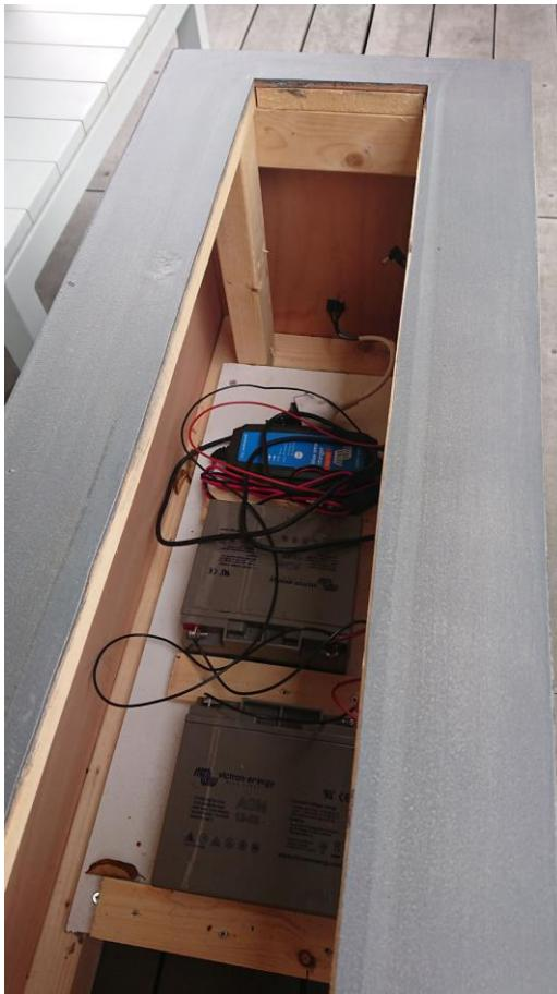
Charging can be done with a battery charger, for example the [Victron Blue Smart](#) charger. The advantage of this charger is that it can be read via a bluetooth connection with your phone - handy if the batteries & charger are hidden away in a place where it is not easy to reach. In the photo on the left you can see both batteries + charger concealed in the mobile box.
